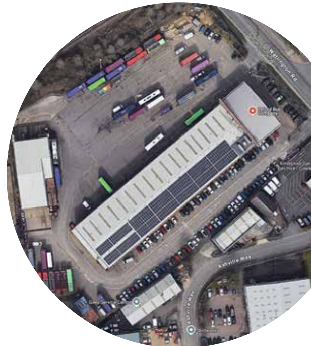
Oxford Bus Company, rooftop solar
