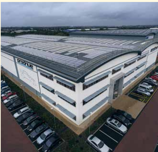
Prodrive, rooftop solar
