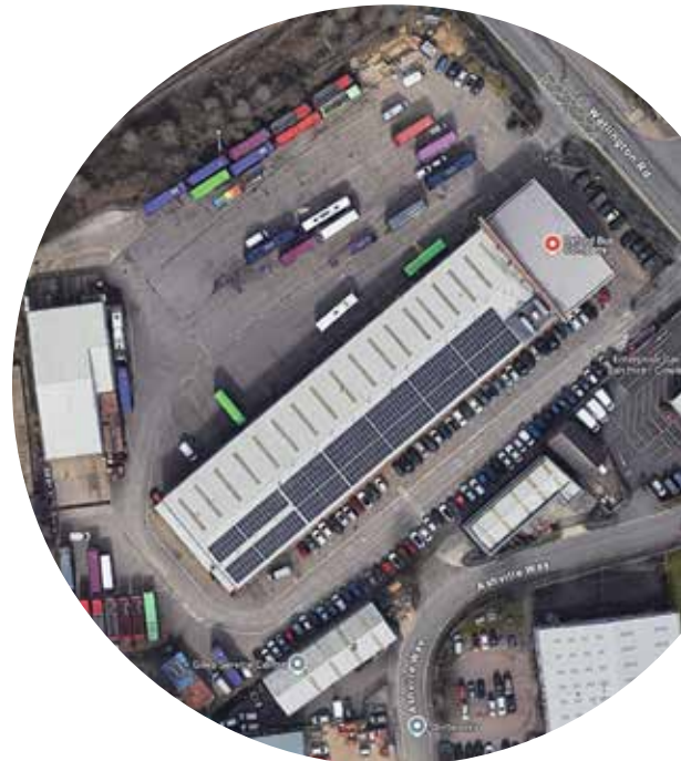
Oxford Bus Company, rooftop solar
