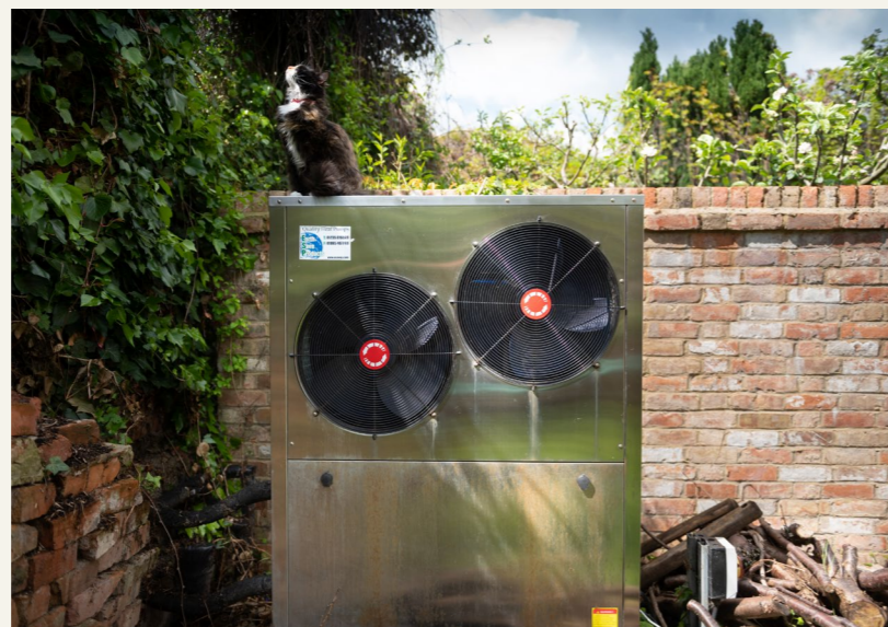
Image 9: Air source heat pump, copyright Low Carbon Hub
