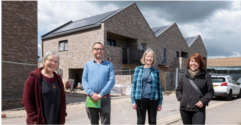
Figure 11: Rose Hill SFN Local Steering Group members with Low Carbon Hub solar PV installation
