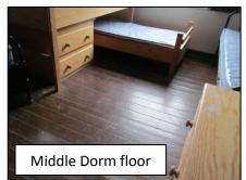
The floor in Middle Dorm is a hung floor over joists with a void below through which heat is lost. There is a constant draught through this floor. If this building is going to be used more during colder months in the future adding insulation will reduce heat loss in winter months, reduce uncomfortable draughts and improve comfort conditions. There are no plans to replace the flooring, however it may be possible to insulate from below as there is a 50-100cm void beneth the building.
