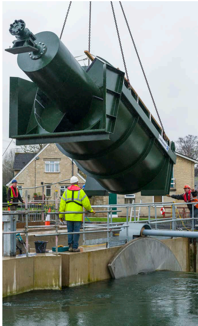
Fitting the Archimedes screw at Osney Lock Hydro (photo courtesy of Andrew Watson)
